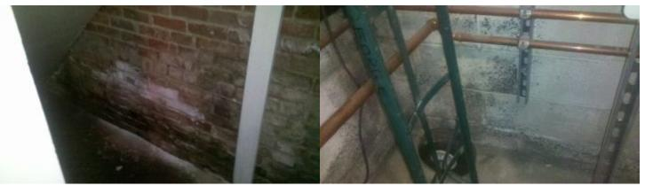
efflorescence and water staining on the foundation
