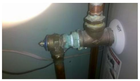
corrosion and short extension on water heater t/p relief valve
