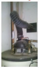
improper flue on water heater
